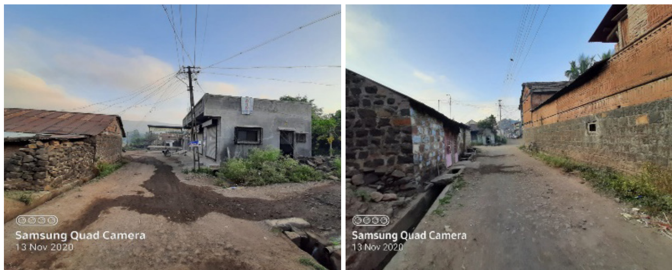
Figure 4: Open Sewage in Gulumb
