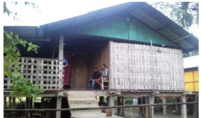
Figure 1: Houses Constructed on Raised Platforms
