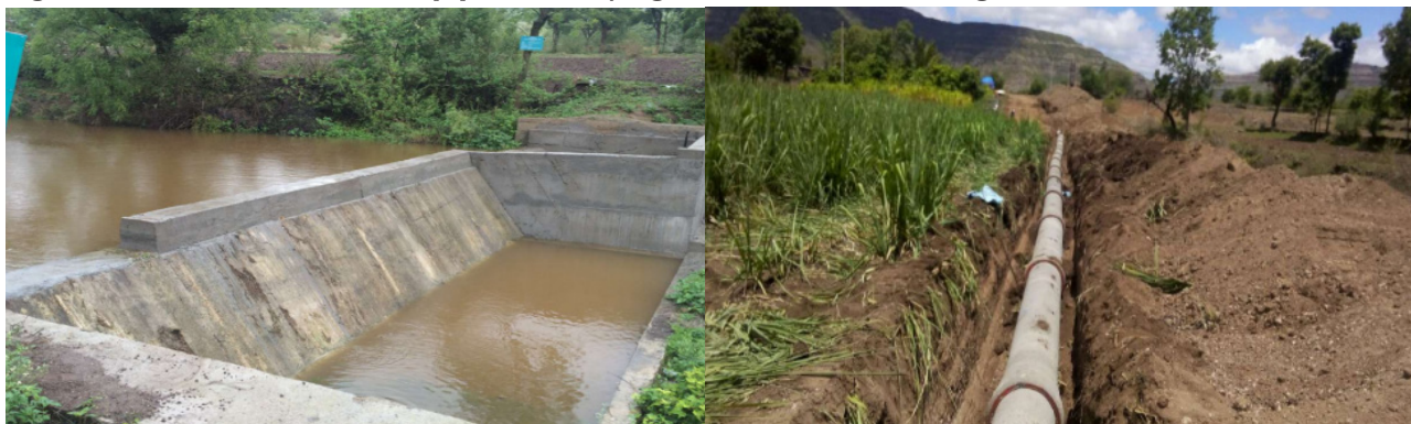
Figure 1: Percolation tank and pipeline carrying water in Gulumb village
