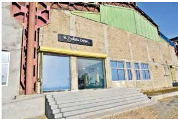
25000 sq. ft. manufacturing plant near Ahmedabad, Gujarat
