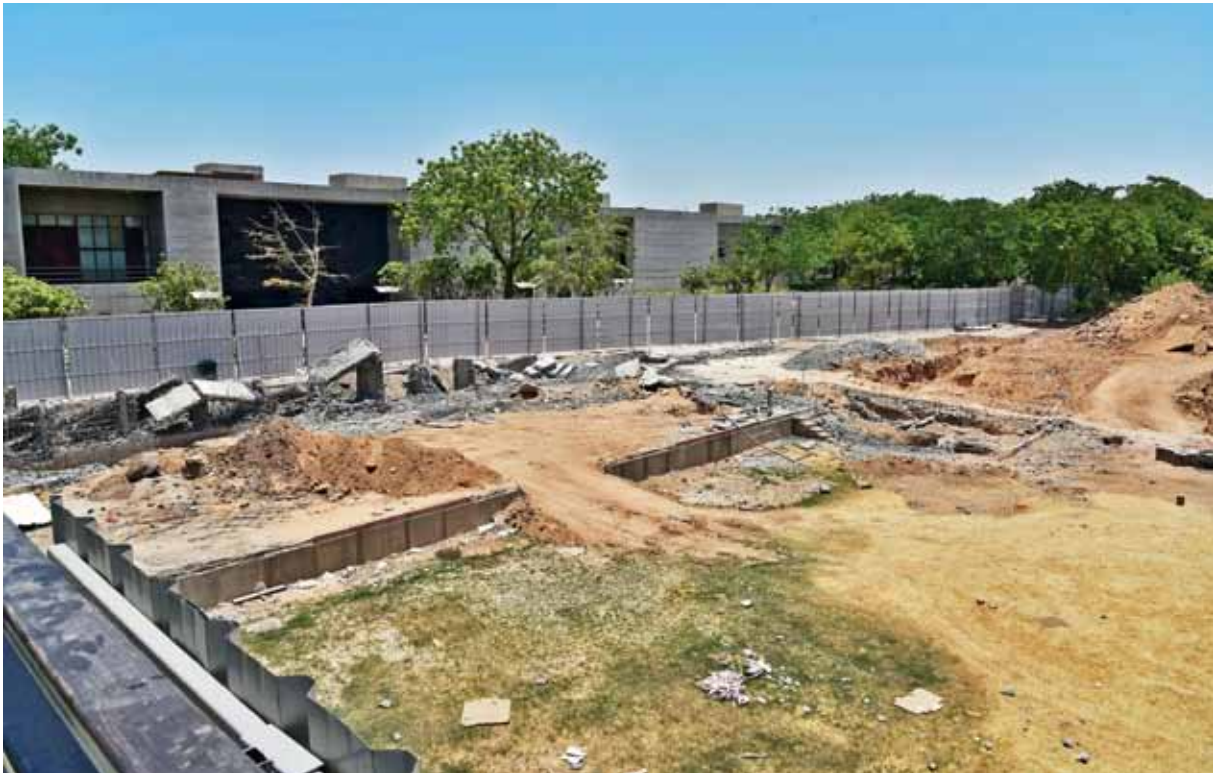
Ongoing construction in the IIMA New Campus
