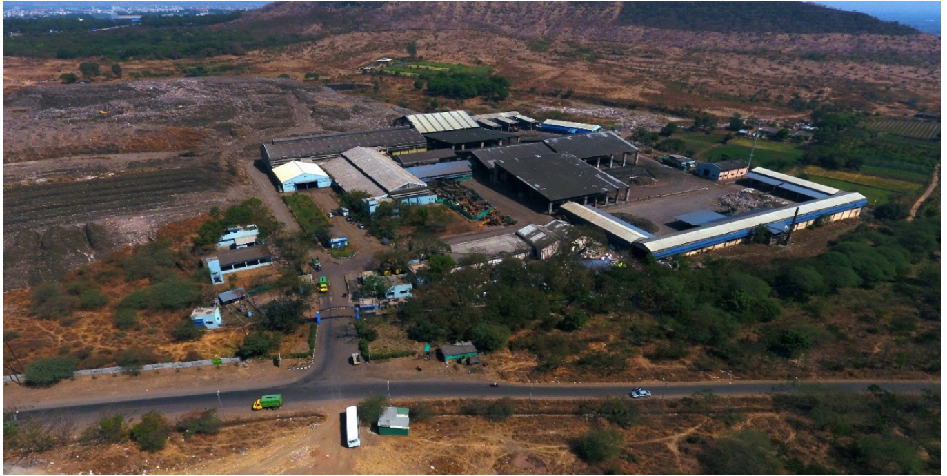
Figure 8: 500 Tons/Day Integrated Solid Waste Management Plant for Nashik Municipal Corporation
