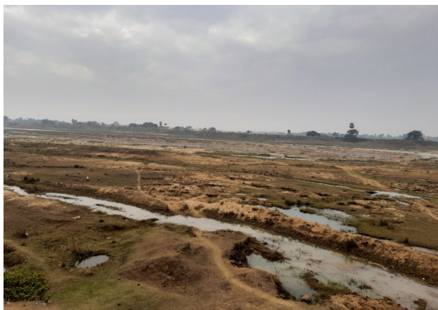
Figure 1: Non-Functional Outlet in Chandan river bed
