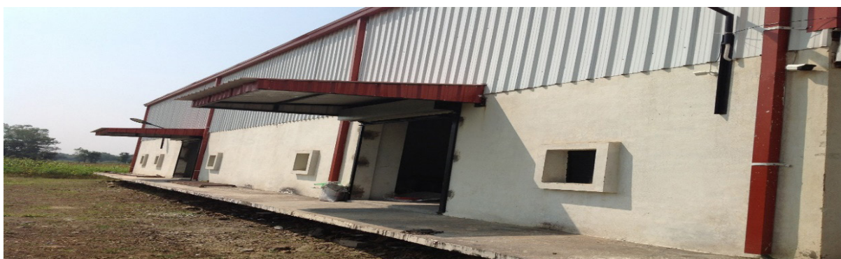
Photo 4.5: Newly constructed modern warehouse of RRPPC
